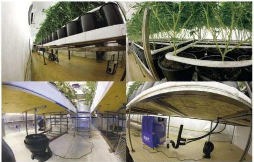
Clockwise: Plant containers on raised tables; a top-feed irrigation system; fans are kept underneath for air circulation; drainage piping for table run-off.
